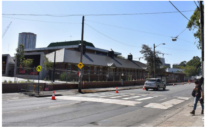
Above: Unshaded concrete and asphalt surfaces in Green Square
