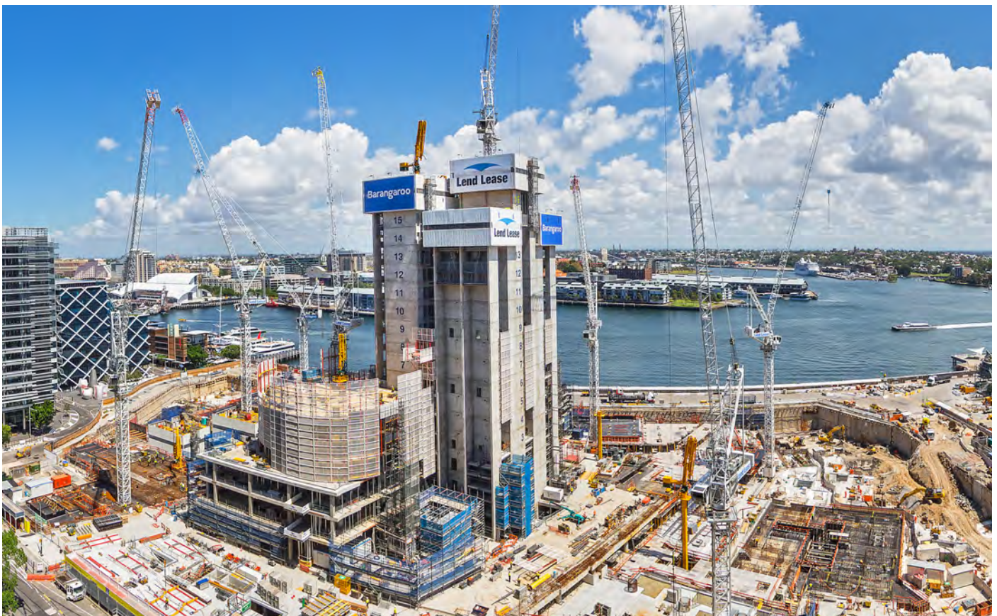
Figure 6: Construction of Barangaroo South
