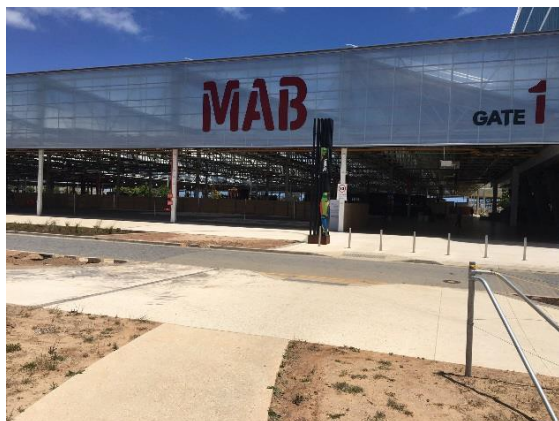
Figure 6 The old Mitsubishi factory in Adelaide, Tonsley, is being developed into an urban innovation precinct and is part of the Adelaide Living Laboratory Hub.
