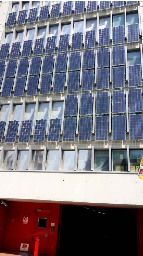
Figure 12: Solar panels as exterior cladding, Barcelona, Spain.
