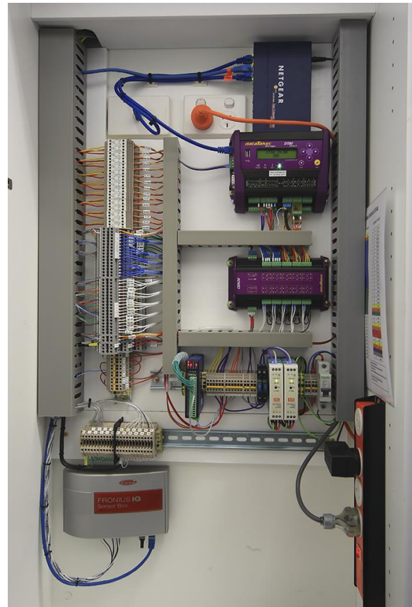
Figure 2: Data logger arrangement at Josh's House in Perth, WA (Photo credit: Morgan Gilham).
