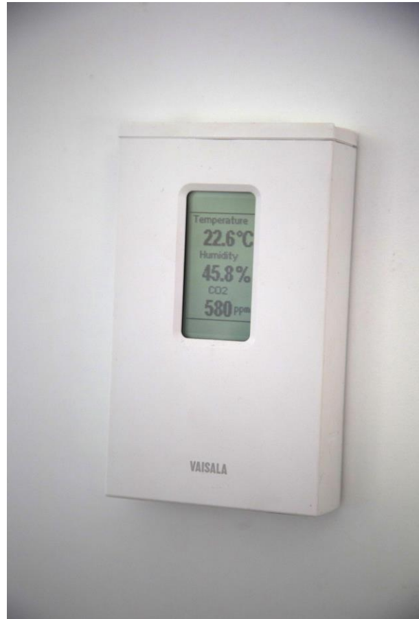
Figure 1: Wall mounted sensor for monitoring temperature, relative humidity and carbon dioxide levels at Josh House in Perth, WA (Photo credit: Darcy Hodgkinson).
