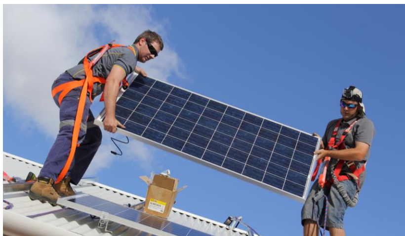
Above: Solar panels being installed.
