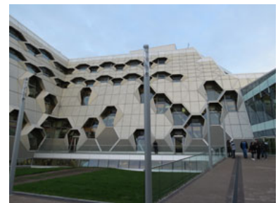
Figure 2 Outside Low impact building, City Lab Coventry.
