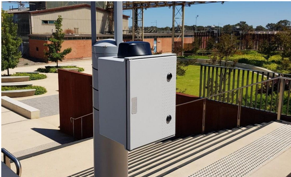
Typical installation example of Addinsight Omnia Capture Station (SAGE Automation, 2019)
