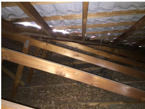
Figure 15. Unsarked gable roof in a residential building in NSW (Source: Munsami 2018)
