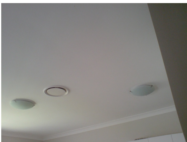
Figure 20. Digital image of a ceiling space (Source: Munsami 2018)
