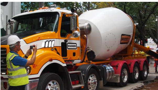
Figure 5. Casting of Geopolymer concrete.
