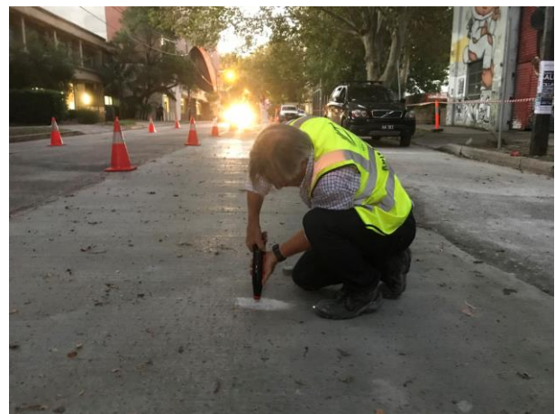
Figure 7. Rebound hammer testing at 27 hours.
