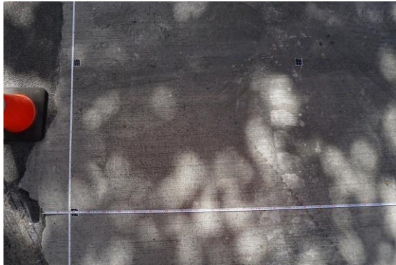
Figure 13. Surveying measurement tapes and photogrammetry targets.
