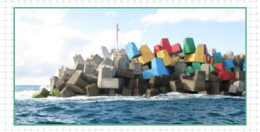
Density is a key parameter in the stability of coastal armour units. It is significant because the armour stability increases with the density cubed, so small increases in density have a significant impact on a structures stability. This has dramatic impacts on both new structures and the maintenance of existing infrastructure.
