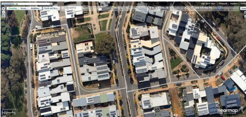
Figure 1 An aerial view of some homes at Lochiel Park.
