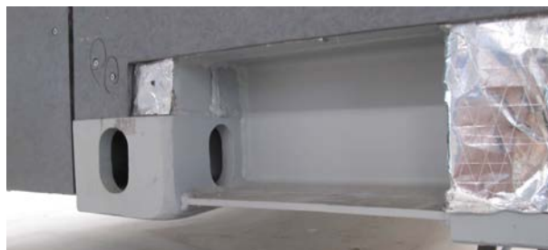
Figure 22 - Detail of the corner casting used for lifting
