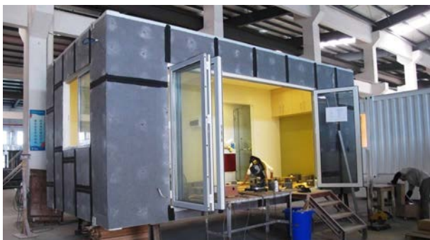
Figure 20 - Second stage of external cladding and work on internal finishes
