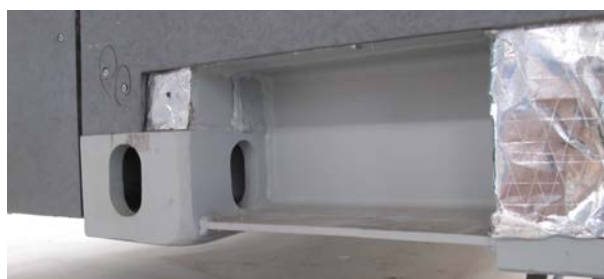
Figure 22 - Detail of the corner casting used for lifting
