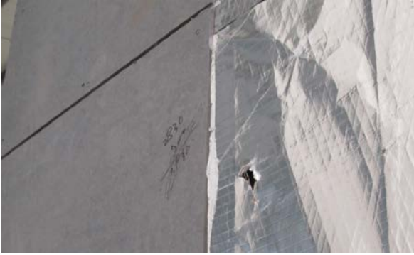
Figure 23 - Cladding waterproofing and openings in membrane
