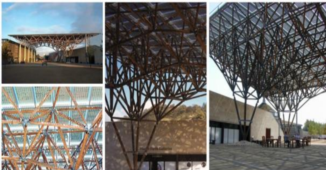
Figure 23: Earth Centre Timber PV structure Source: Carpenter Oak & Woodland; Terry Miller
