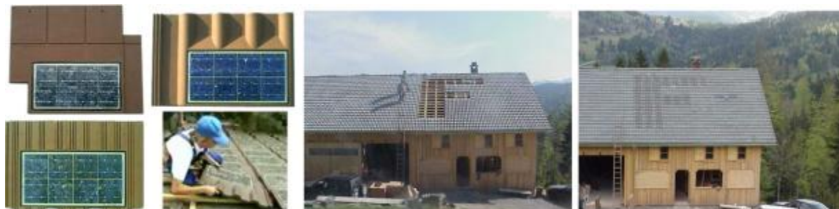
Figure 14 – STEPdesign solar roof tile on clay tile
