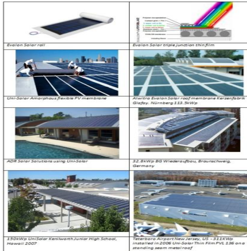
Figure 30: Flexible PV membranes on metal roofs
