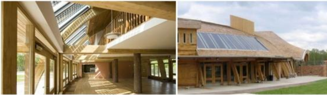
Figure 24: Shorne Wood Country Park (UK) PV integrated within a timber shingle roof
