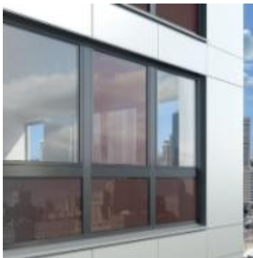
Figure 37: Schüco ProSol TF+ multi-layer a-Si translucent PV cladding materials
