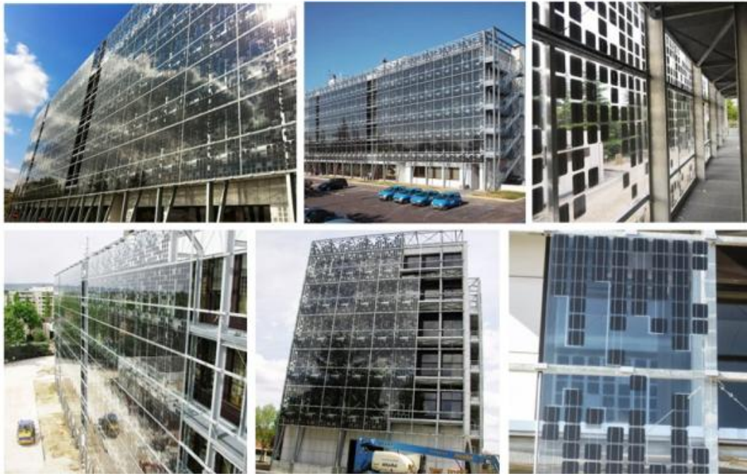
Figure 48: GDF Suez, Solal Building Dijon Source: Philéas Atelier d'Architecture, 2011
