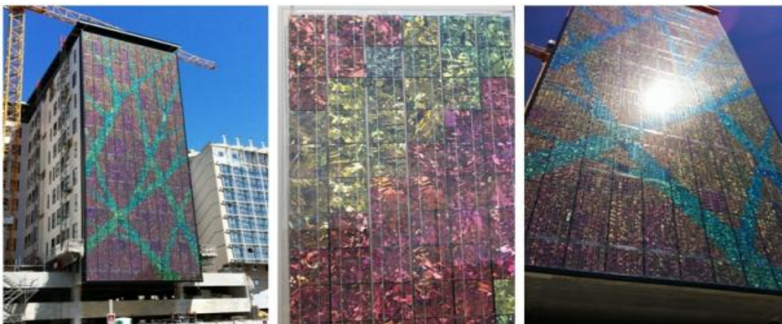
Figure 46: BIPV poly-crystalline façade La CUB – Bordeaux, France
