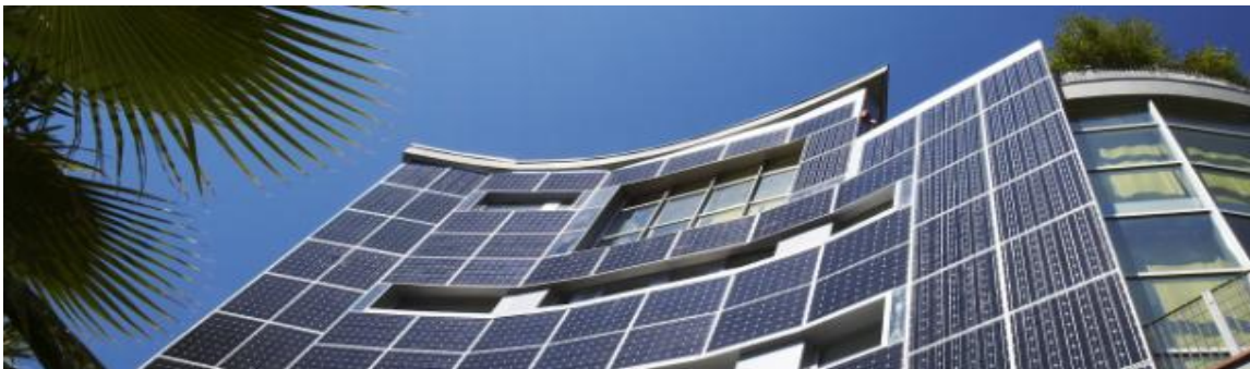
Figure 45: Conventional panels cleverly integrated into a building façade
