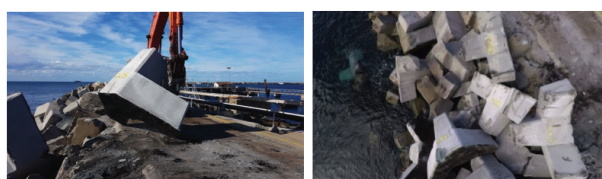
(e) Placement of Hanbar units on breakwater
