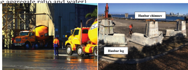
(a) Batching at Cleary Brothers plant, Port Kembla
