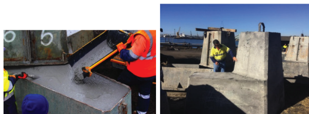
(c) Concrete pouring and compaction
