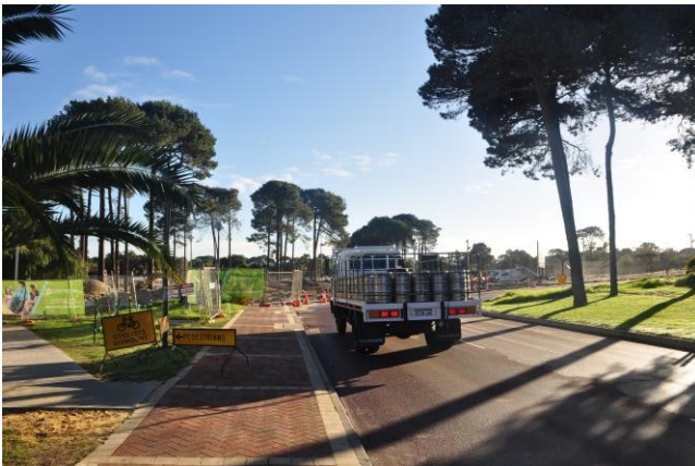
Figure 1: Greater Curtin redevelopment underway
