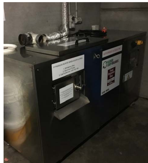
Fig 1: Closed Loop composter being installed at Swinburne University, Melbourne (Sep 2016).
