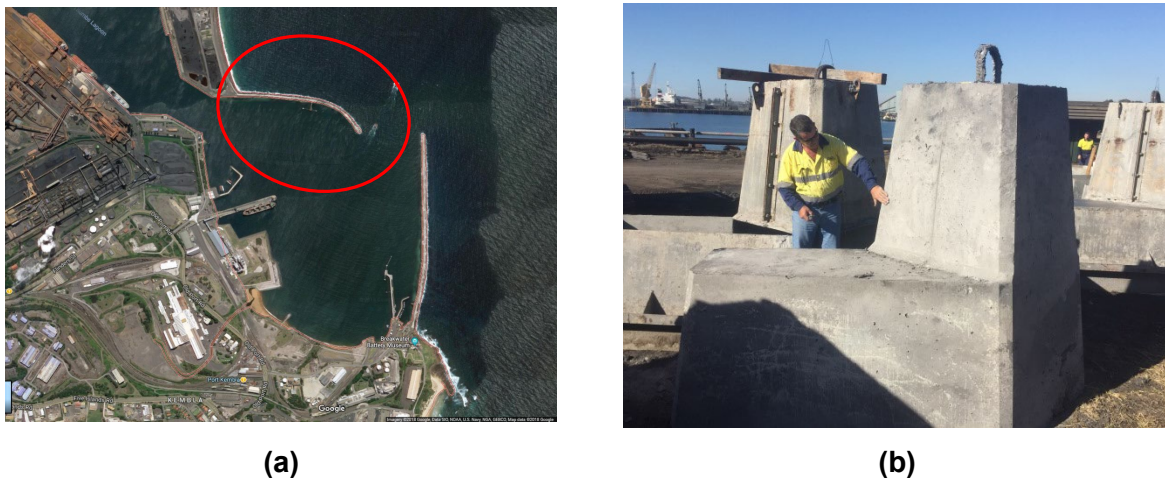
Fig. 6.1. High-density GPC (a) site location- Port Kembla northern breakwater (Google maps) (b) GPC Hanbar Armour Unit.
