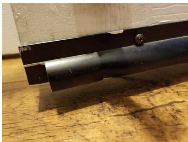
Figure 3.4 To reduce air leakage, fit external doors and windows with weather strips (left) and self-adhesive foam (right).
