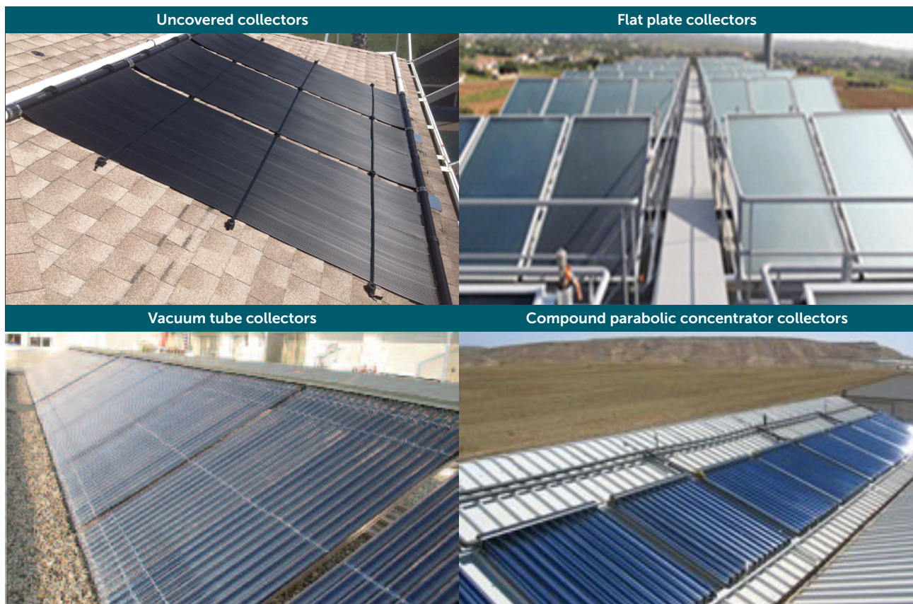
Figure 3.1 Types of solar thermal collectors.
