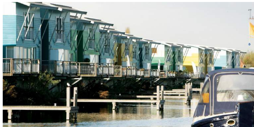
Amphibious buildings and the mooring posts (Maasbommel, The Netherlands) Figure 18: Amphibious buildings (atelier GROENBLAUW)
