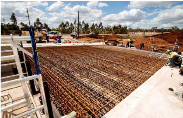
Figure 66. Reinforcement Installation at Toowoomba Bridge Site, QLD in September 2014 (Wagners).
