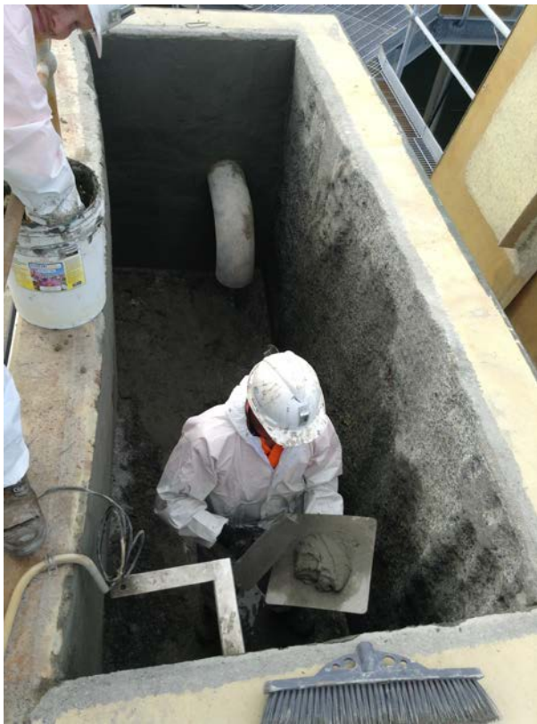
Figure 122. Application of Miliken's mortar (Geospray) to repair the deteriorated surface drain.
