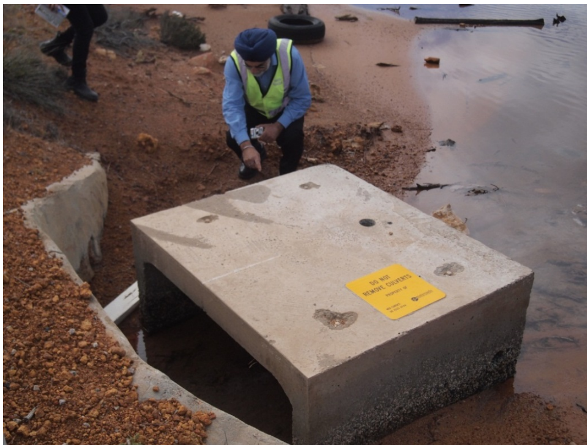
Figure 21. Geopolymer concrete culvert at Lake King site, WA, in October 2015.
