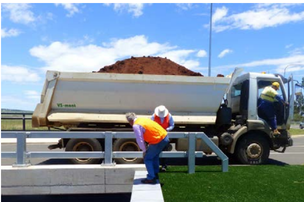
Figure 80. Live load testing: truck position 3.
