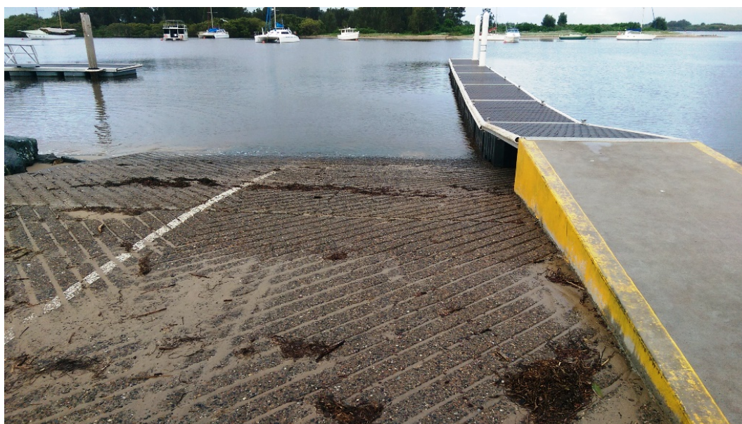
Figure 99. Site view of Westport boat ramp project at Port Macquarie, NSW.
