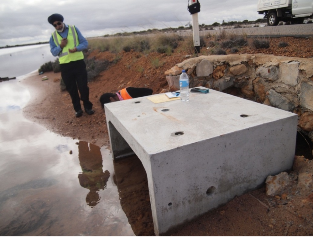
Figure 22. OPC concrete culvert at Lake King site, WA, in October 2015.
