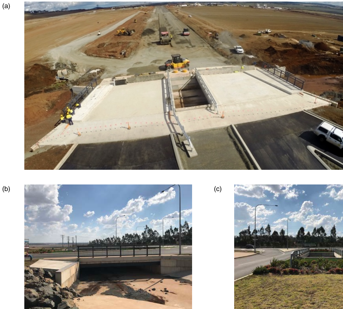
Figure 64. (a) Geopolymer concrete bridge at Wellcamp airport business park precinct, Toowoomba Queensland: (a) nearing completion at in in September 2014 (photo courtesy of Wagners); (b)-(c) completed bridge and road development (photo taken August 2017).
