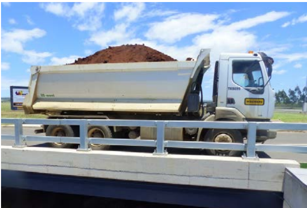
Figure 79. Live load testing: truck position 2.
