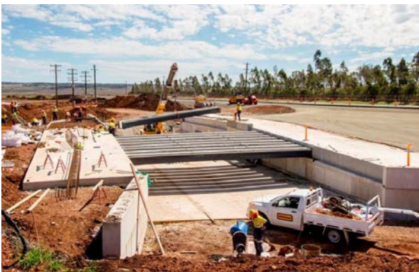
Figure 67. Installation of FRP Girders at Toowoomba, QLD, in September 2014 (Wagners).
