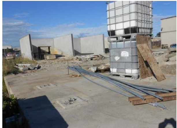
Figure 2. Main slab at Campbellfield site, VIC in March 2015.
