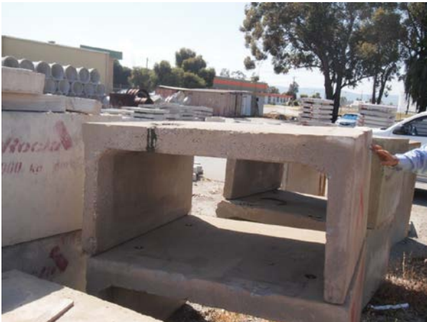
Figure 42. Geopolymer concrete culvert at casting yard in Perth, WA, in October 2015.
