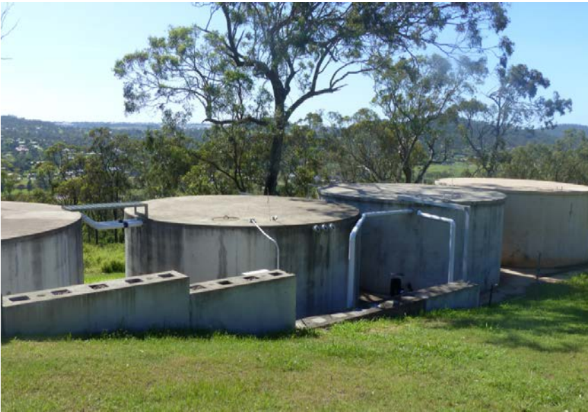
Figure 13. Geopolymer and OPC concrete water tanks at Toowoomba site, QLD, in December 2015.
