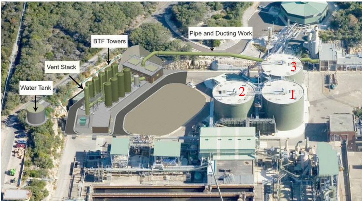
Figure 5. Aerial view of North Head Wastewater Treatment Plant showing digesters 1 to 3.
