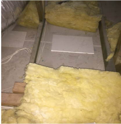
Figure 13: Displaced insulation in BASIX-compliant dwellings with high space heating and cooling energy consumption (Munsami, 2019)
